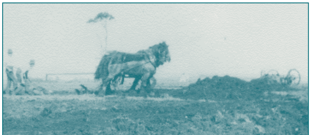
^ WARRAGUL GOLF COURSE UNDER CONSTRUCTION Reproduced with permission of Warragul Historical Society
